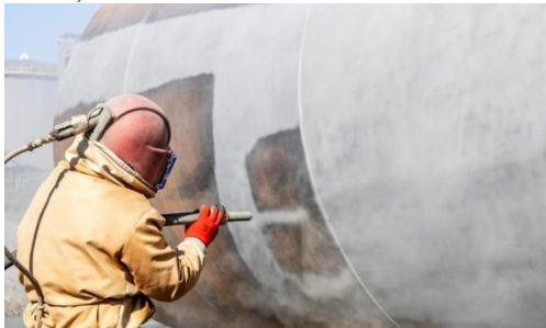
Gambar 1. Proses Sandblasting
