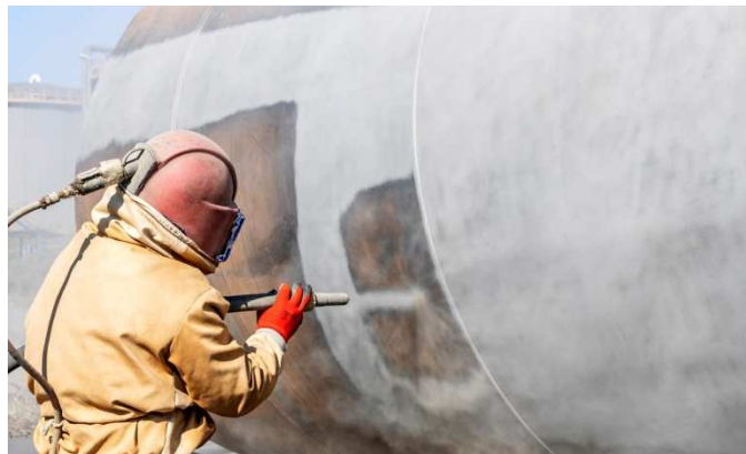
Gambar 2.1 Proses Sandblasting Sumber : (Bangun dkk, 2017)
