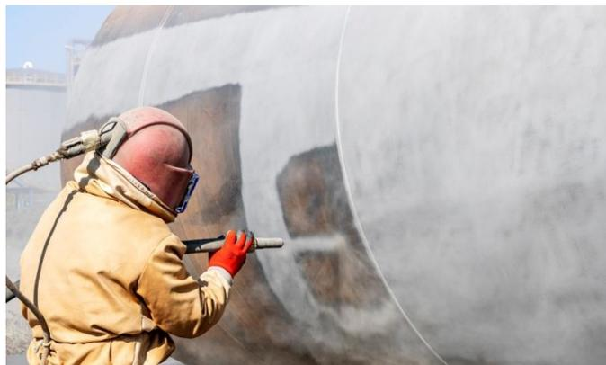
Gambar 2.1 Proses *Sandblasting*
