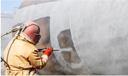
Gambar 1. Proses Sandblasting
