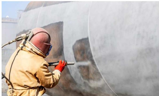
Gambar 2.1 Proses *Sandblasting*
