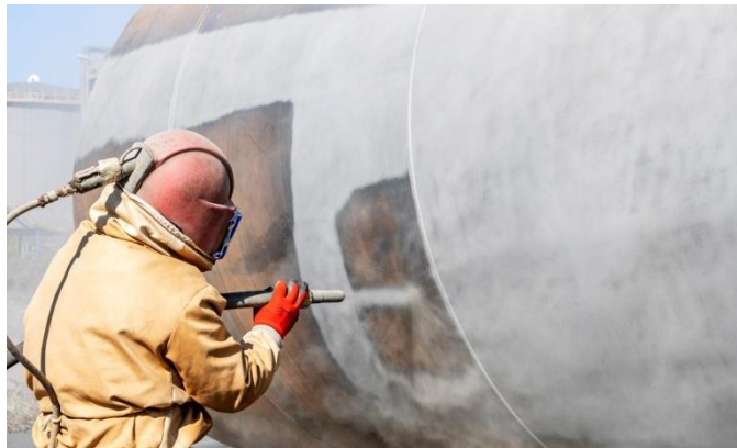
Gambar 2.1 Proses Sandblasting
