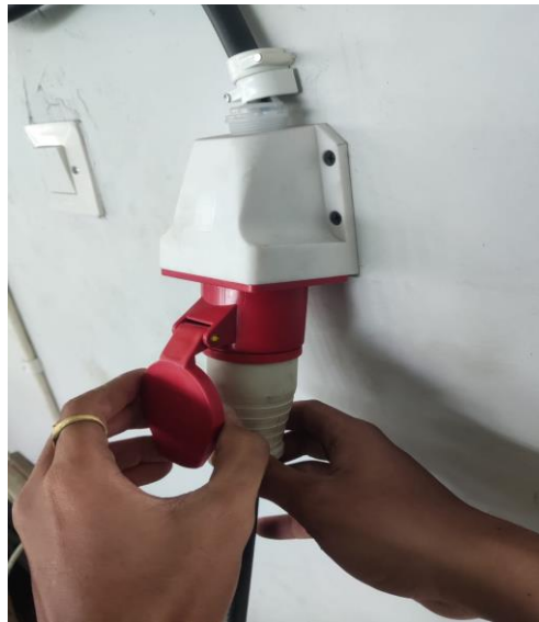
Gambar 3.9 Pasang stop contact
