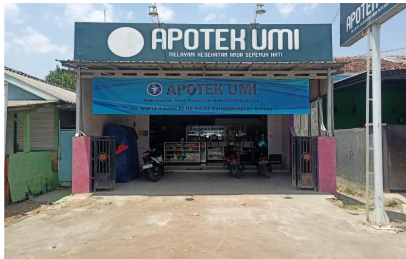
Gambar 2.1 Gedung Apotek Umi
