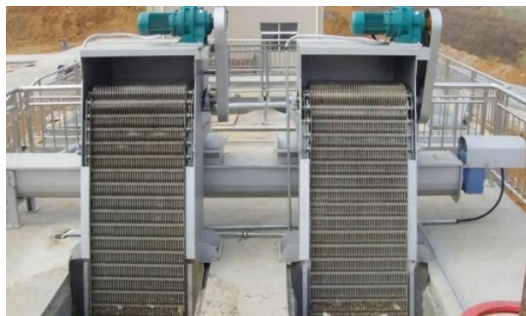
Gambar 2.3 Mechanical Bar Screen (Bioetp, 2024)
