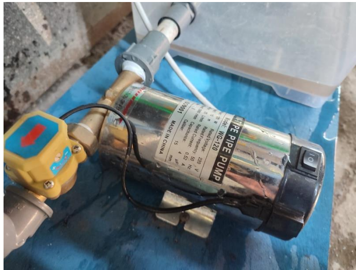
Gambar 3. 15 Pompa Booster
